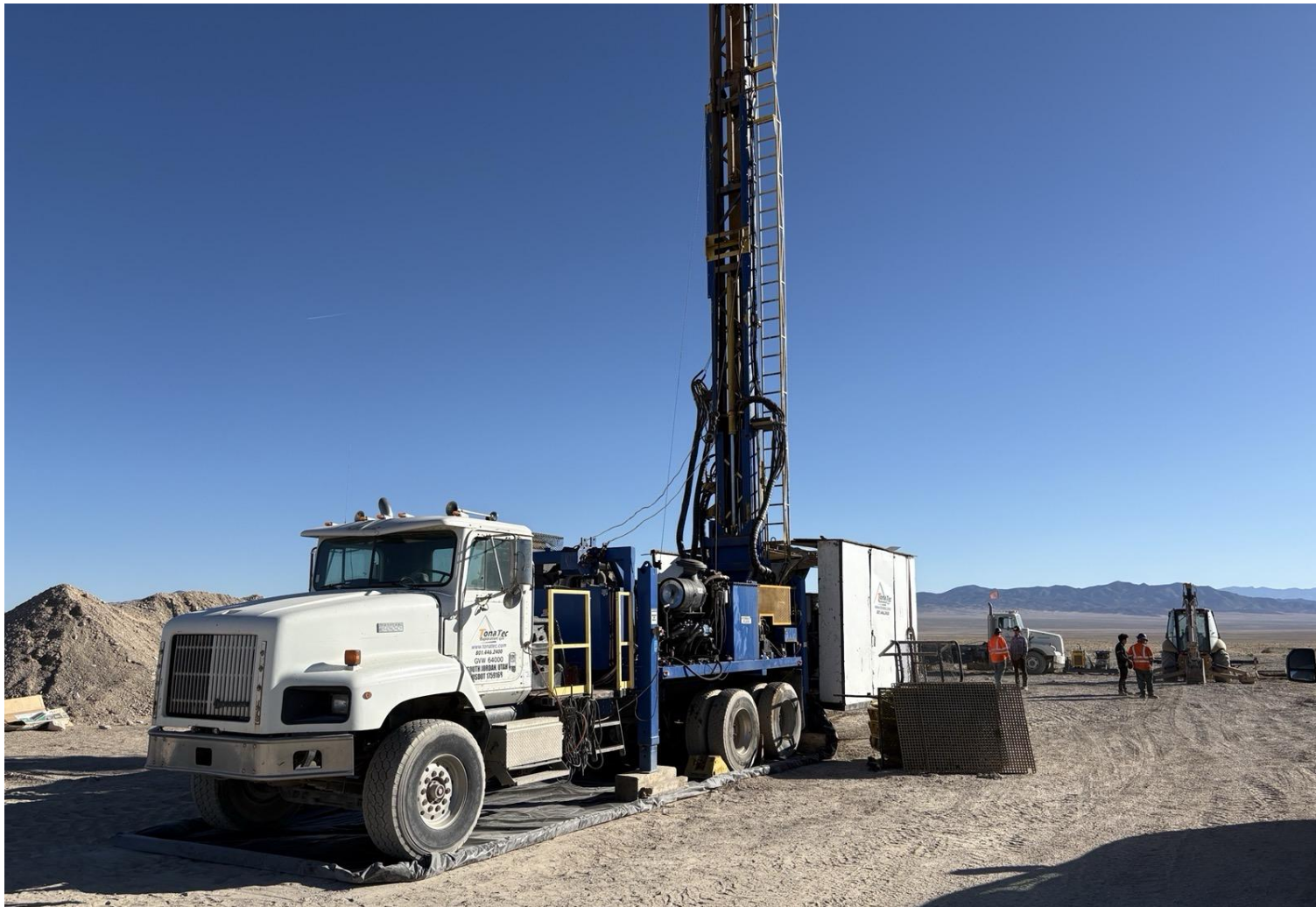
Figure 4. TonaTec diamond drilling rig in action
